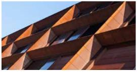
COR-TEN® and S355JOWP are structural steels with a minimum yield strength of 345-355 MPa, alloyed with Phosphorus (P), Silicon (Si), Copper (Cu), Chromium (CR) and Nickel (Ni). Because of this alloying, the surface of COR-TEN® A and/or S355JOWP will, under the influence of varying wet and dry atmospheric conditions, form an oxide layer called patina. This patina completely seals-off the steel surface from the atmosphere and thus forms a corrosion-resistant coating. Both beautiful and durable!
